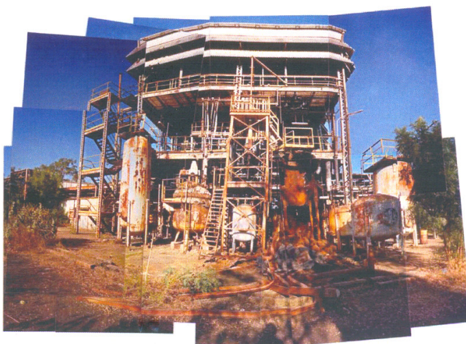
Abandoned Union Carbide Plant, Bhopal India 2005
