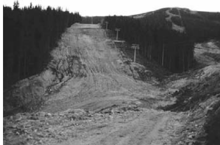
Erosion on the ski slopes outside of the skiing season
